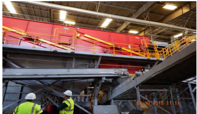
Conveyor system at recycling plant.
